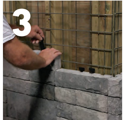
Attach Tandem Veneer with Connector
