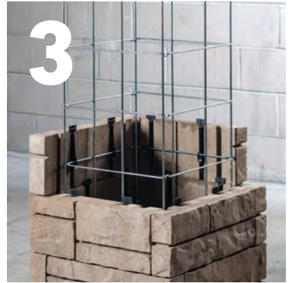
3 Repeat step 2 and fill with ¾" crushed rock until column is complete
