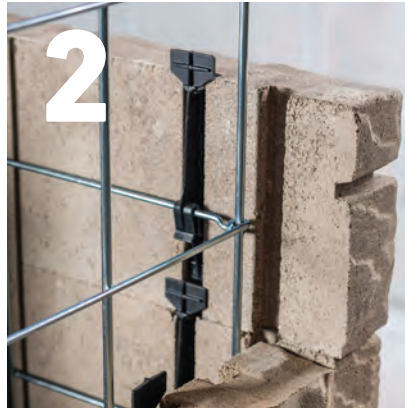
2 Use connector to attach Ashlar Tandem Veneers to grid
